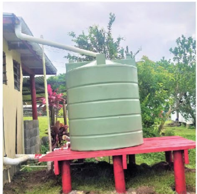
↑↑ The above picture depicts the completed secondary water sources installed in Rokovuaka ECE with proper tank stand. The tank is connected to the gutter for rain water harvesting during rainy season and it is also connected to the main water supply line to automatically fill in the tank once empty. Photo Credit: Save the Children Fiji
