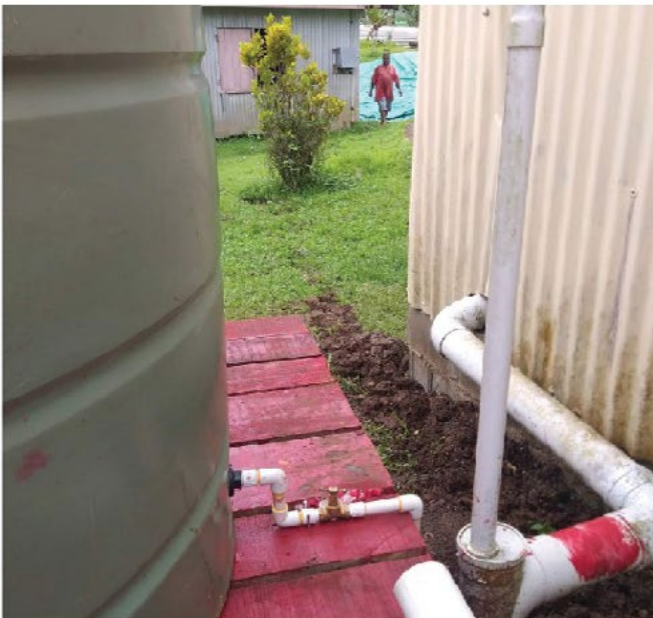
↑↑ The above picture depicts the completed secondary water sources installed in Rokovuaka ECE with proper tank stand. The tank is connected to the gutter for rain water harvesting during rainy season and it is also connected to the main water supply line to automatically fill in the tank once empty. Photo Credit: Save the Children Fiji
